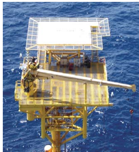
High Island A-442 single well caisson structure shows limited deck space. (All graphics courtesy of Maritech)
